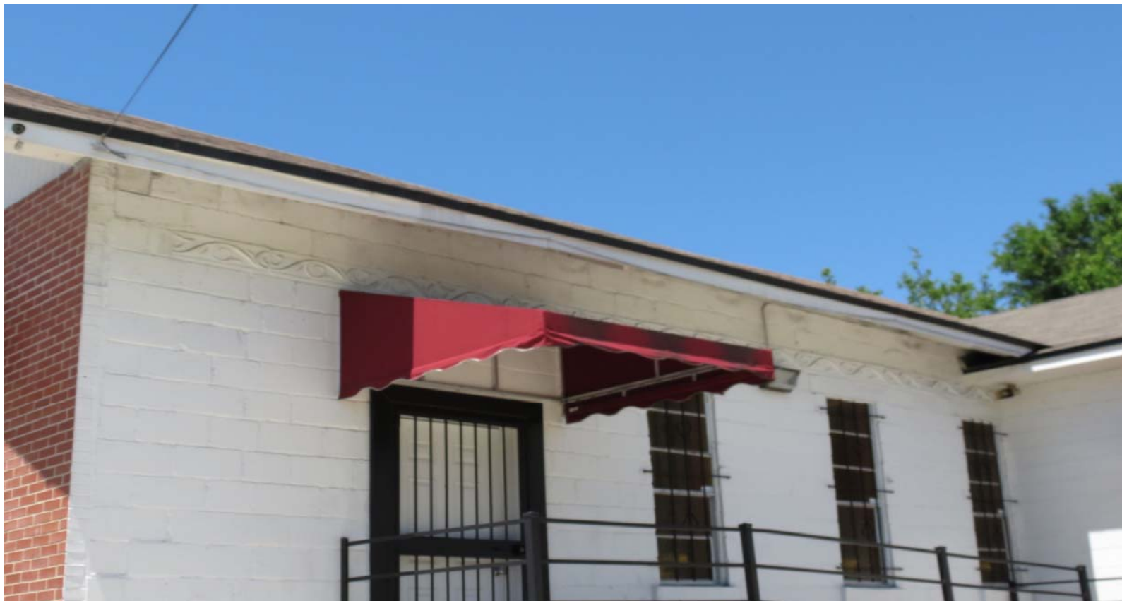
LM-19-01 ALLEN CHAPEL A.M.E. CHURCH 1529 SWAN STREET PHOTO # 24 APRIL 17, 2018
