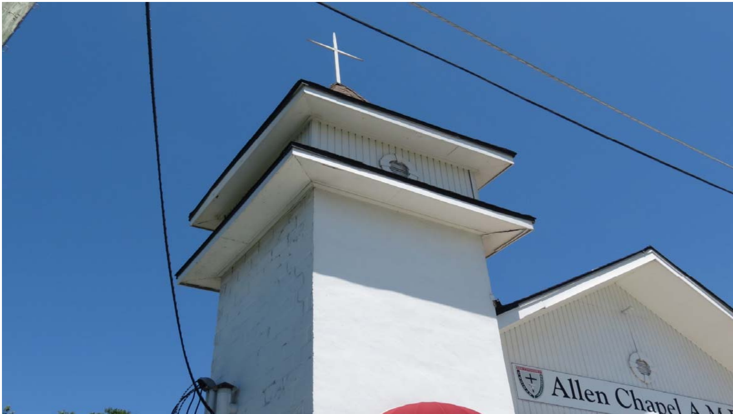
LM-19-01 ALLEN CHAPEL A.M.E. CHURCH 1529 SWAN STREET PHOTO # 14 APRIL 17, 2018
