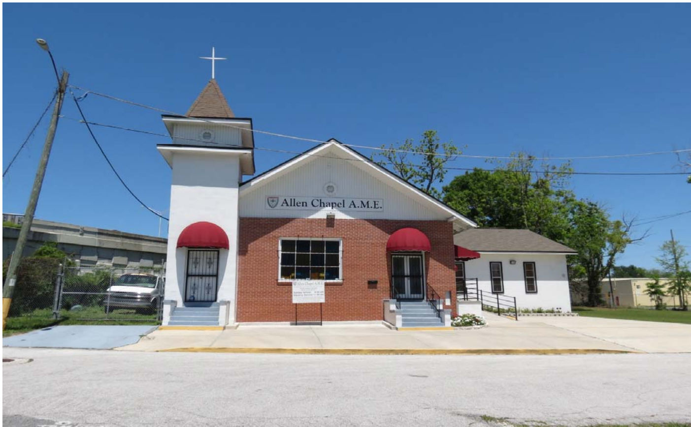
LM-19-01 ALLEN CHAPEL A.M.E. CHURCH 1529 SWAN STREET PHOTO # 10 APRIL 17, 2018
