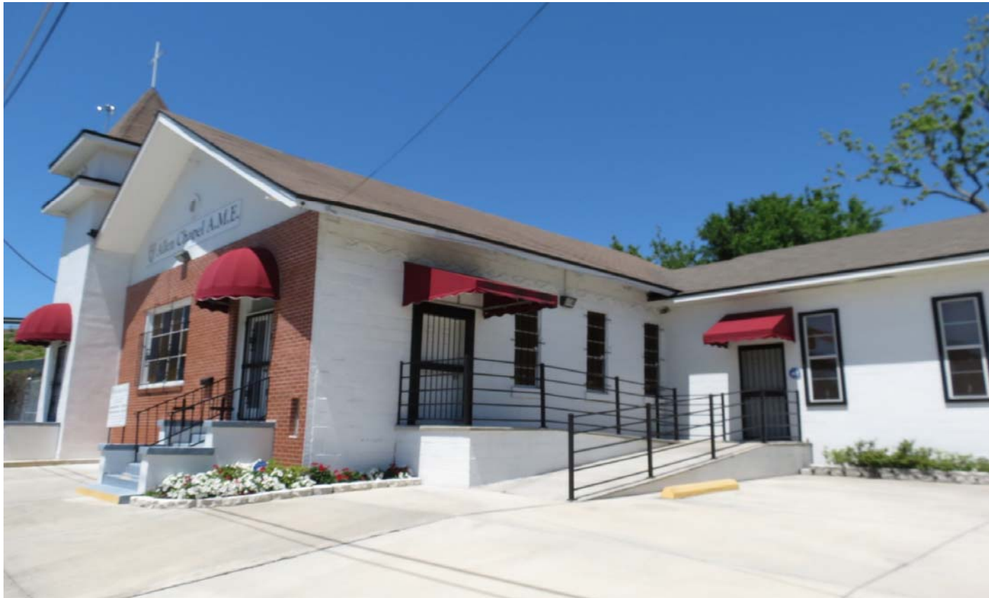
LM-19-01 ALLEN CHAPEL A.M.E. CHURCH 1529 SWAN STREET PHOTO # 22 APRIL 17, 2018
