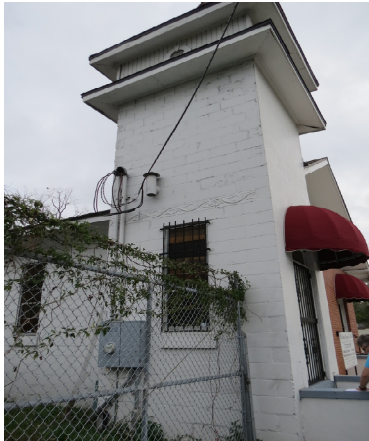
LM-19-01 ALLEN CHAPEL A.M.E. CHURCH 1529 SWAN STREET PHOTO # 11 JANUARY 4, 2019
