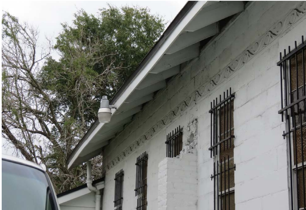
LM-19-01 ALLEN CHAPEL A.M.E. CHURCH 1529 SWAN STREET PHOTO # 32 JANUARY 4, 2019
