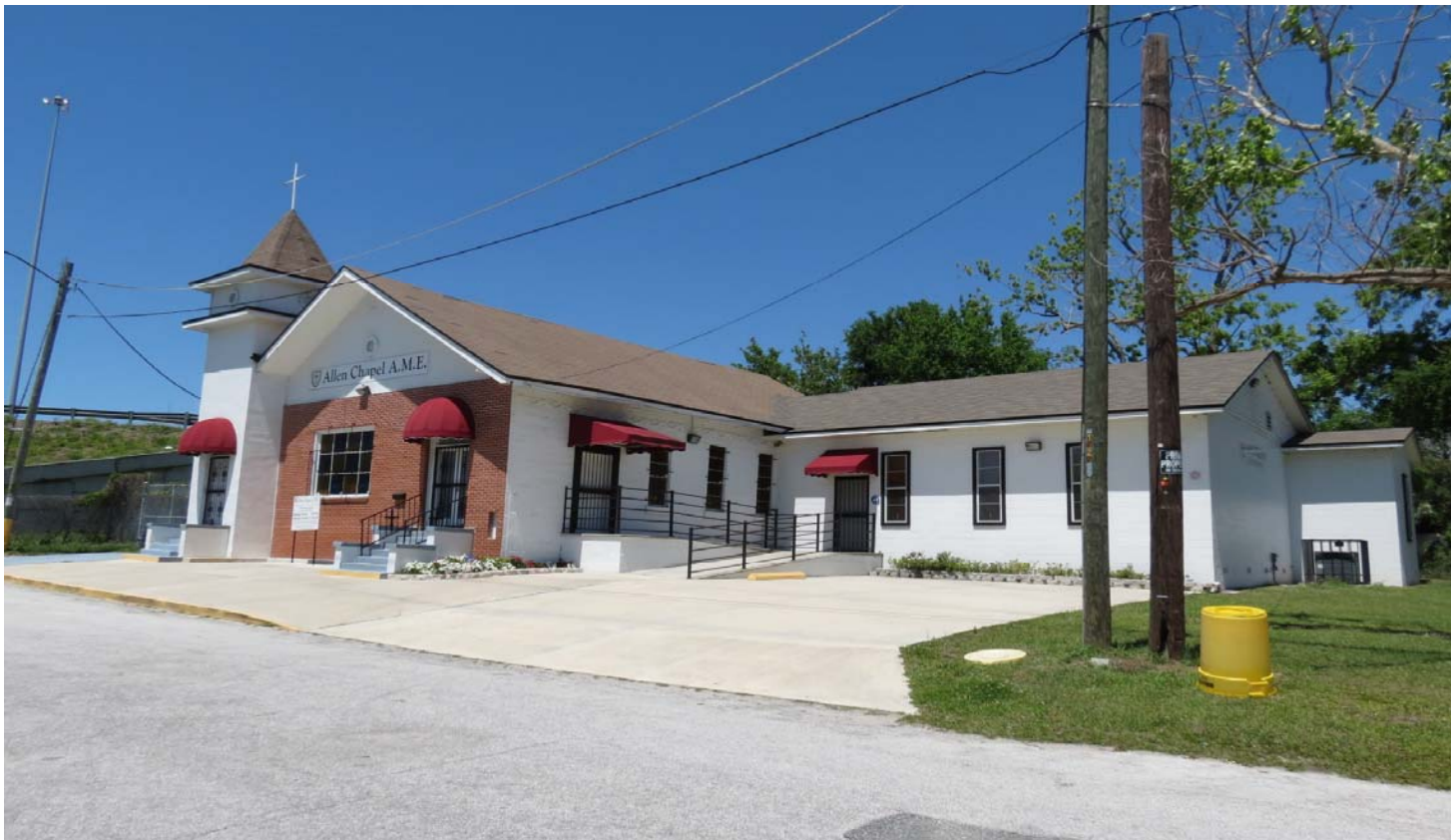
LM-19-01 ALLEN CHAPEL A.M.E. CHURCH 1529 SWAN STREET PHOTO # 8 APRIL 17, 2018
