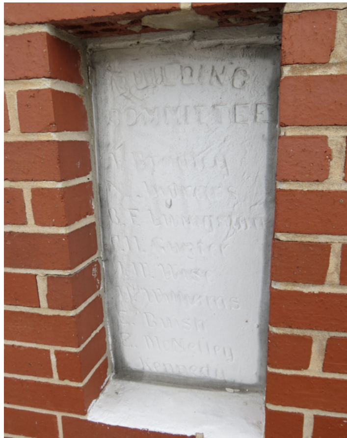
LM-19-01 ALLEN CHAPEL A.M.E. CHURCH 1529 SWAN STREET PHOTO # 21 JANUARY 4, 2018
