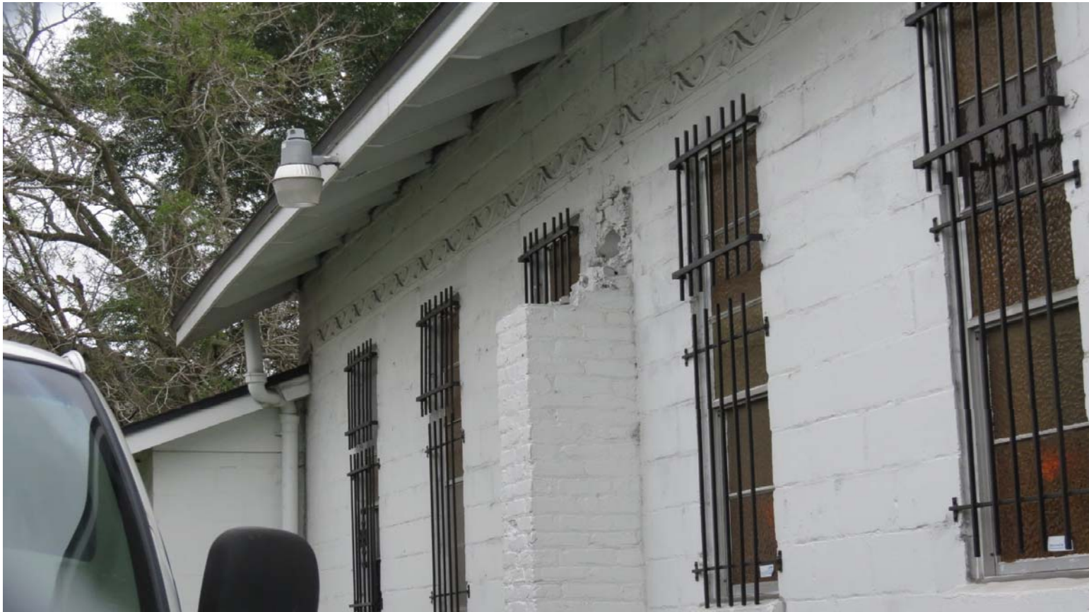
LM-19-01 ALLEN CHAPEL A.M.E. CHURCH 1529 SWAN STREET PHOTO # 33 JANURARY 4, 2019
